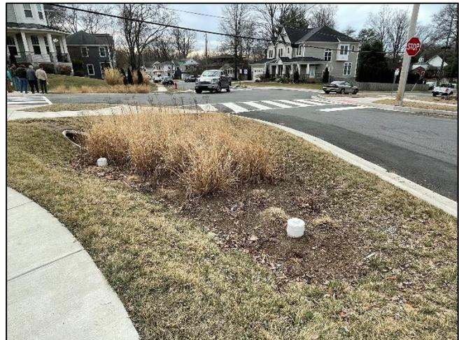
*Bioretention incorporated into traffic calming project.*
