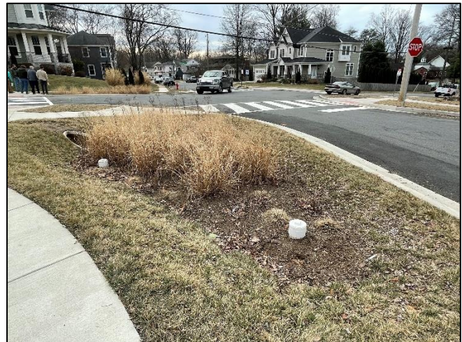
Bioretention incorporated into traffic calming project.
