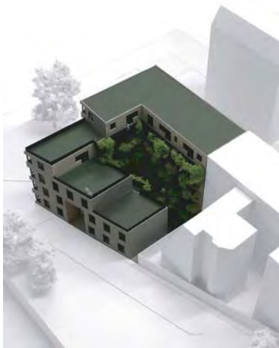
Building step-backs, or decreases in building height, are one neighborhood protection standard. In this example, the building modules on the back of the building are shorter than the ones in front. Neighborhood protection standards would require these shorter heights on the side of the building abutting single-family development.
